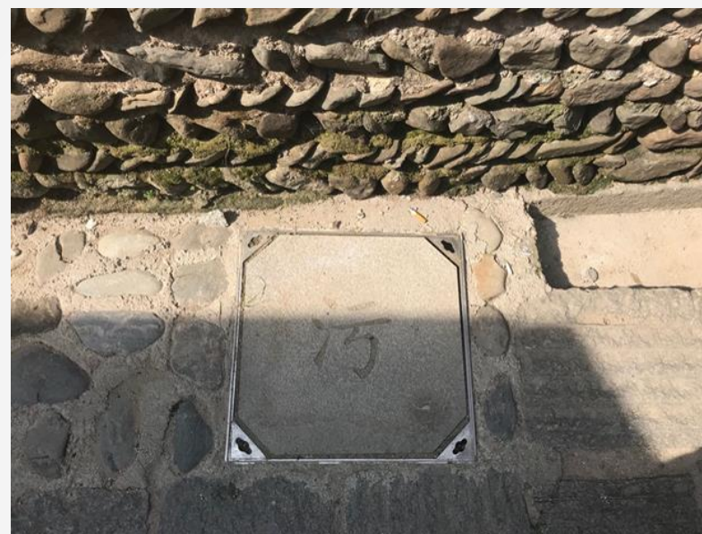
Newly built sewage pipe manhole cover
